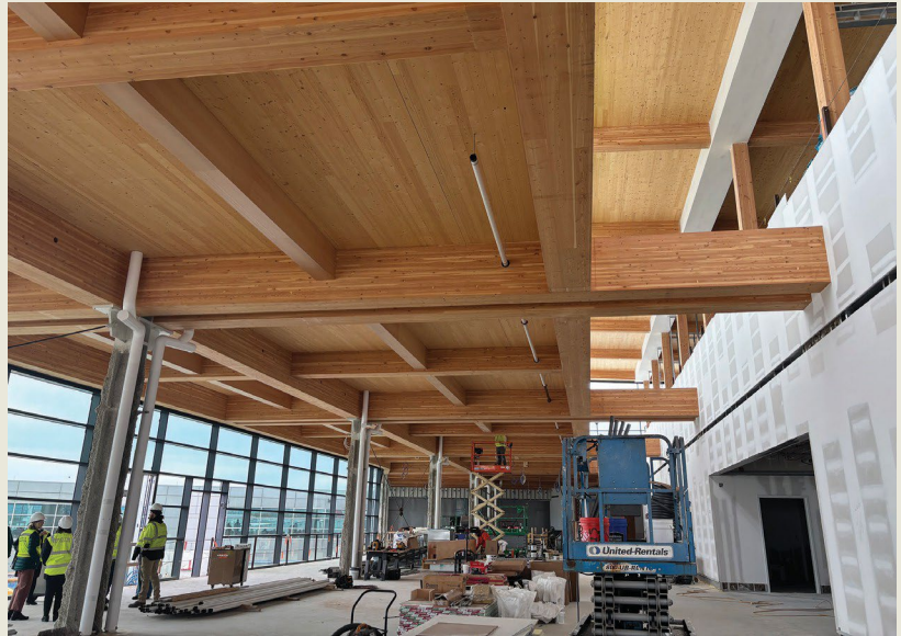
Project in Progress: Patrick Leahy Burlington International Airport in Burlington, VT
