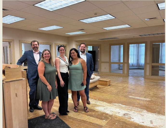
Project In Progress: Gorham Community Learning Center (GCLC) childcare center renovations in Gorham, NH.
